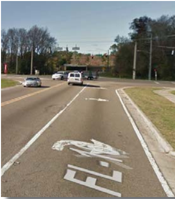
State Road 16 approaching U.S. 17 Intersection
